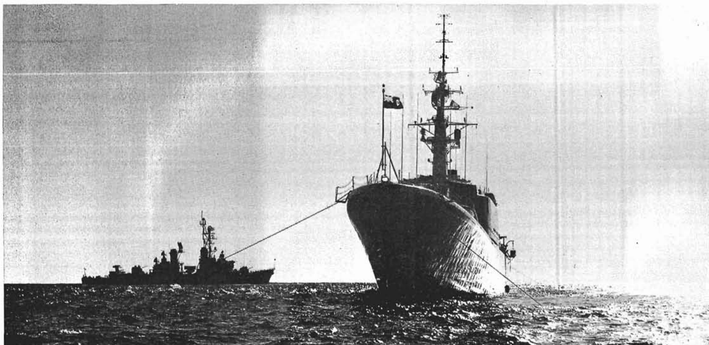
Steadied in position by mooring lines, HMCS Fraser awaits the impact of the blast from a 500-ton TNT explosion during tests in Hawaiian waters early this year. (O-19530-79)
