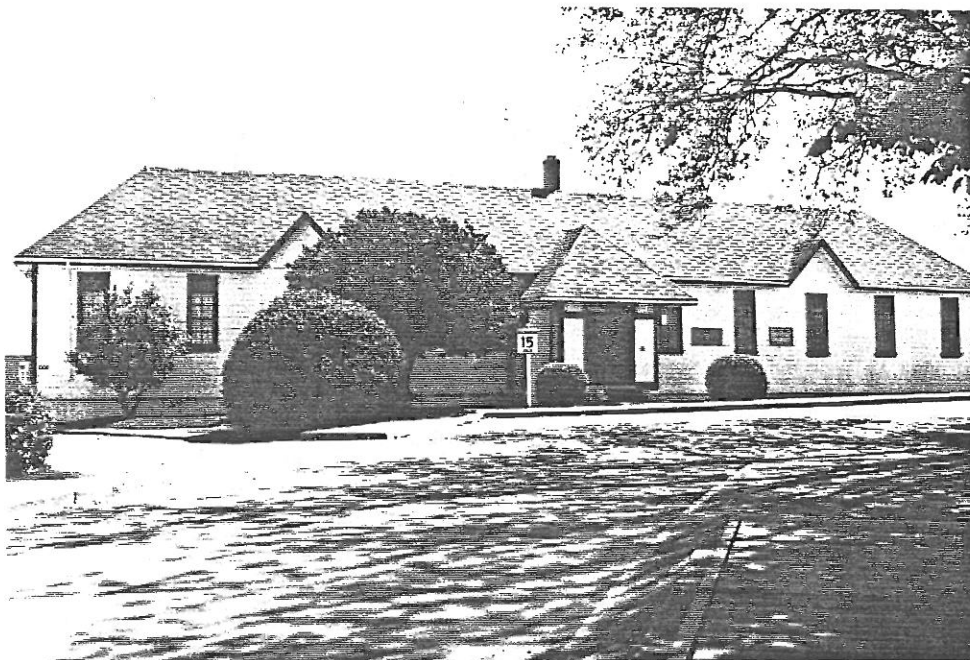
2 Building 1004, main (west) elevation. ( Ian Doull, AHB, Parks, 1989. )
