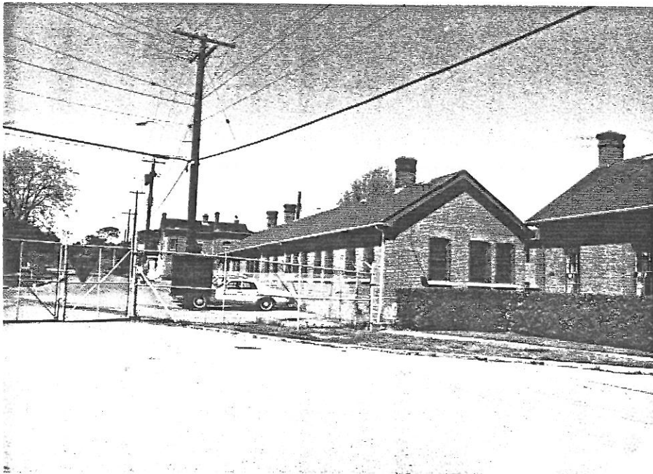
3 Building 1070, rear (south) and end (east) elevations; building no. 1068 is visible at left, no. 1071 stands at right. ( Edward Mills, AHB, Parks, 1989. )
