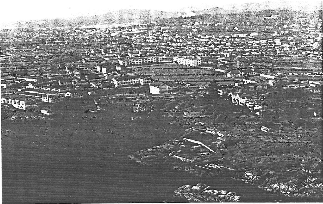
13 Work Point Barracks, looking northwest, 1964. ( Canadian Forces Photo Unit. )
