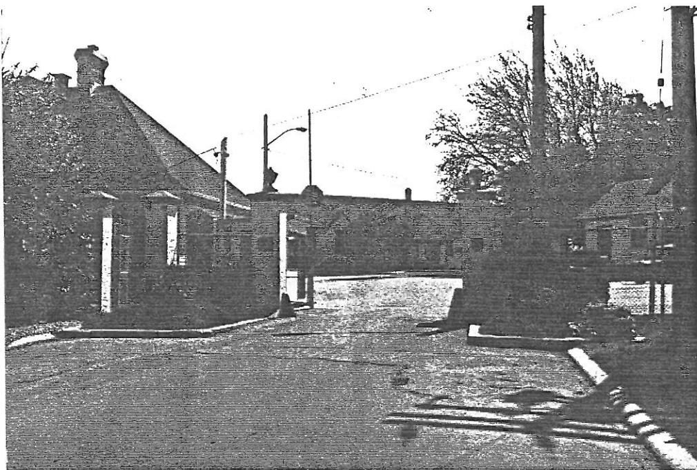
9 Buildings 1001, 1004, 1087 (L-R), looking east through the main gate. ( Ian Doull, AHB, Parks, 1989. )
