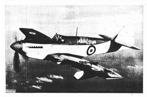
This is the Firefly V with which 825 Squadron, now in the United Kingdom, is being equipped. The squadron will return to Canada February 23 on board H.M.C.S. "Magnificent". An all-metal, two-seat monoplane, the Firefly V is powered by a Rolls Royce Griffon engine. It is equipped with four 20-mm. cannon, radar and radio installations, and the latest airborne anti-submarine devices.
