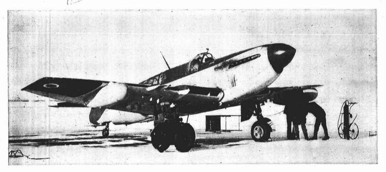
Cold starting tests being carried out on the Firefly 4 at Watson Lake. When the mercury is out of sight, this is not the pleasantest of work.
