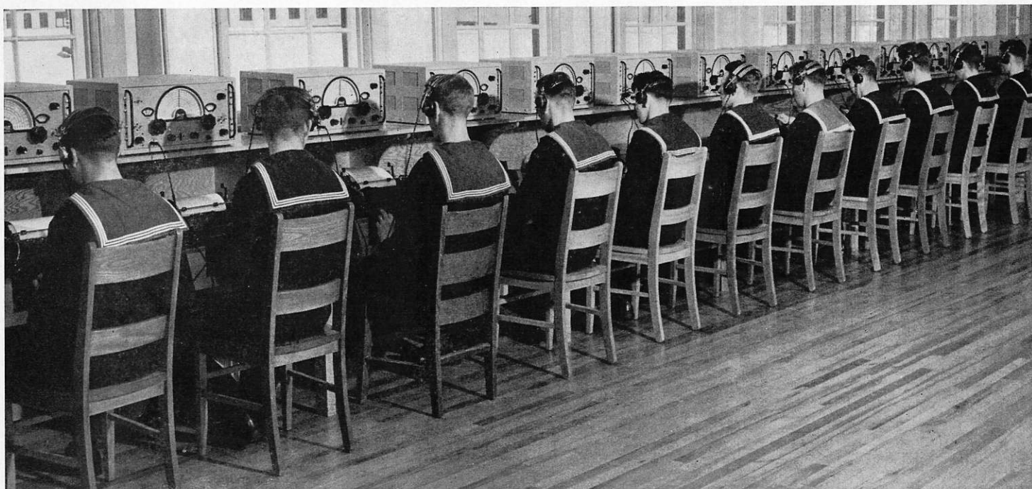
Fifty-three men can be accommodated at one time in the instructional receiving room, used for training basic classes in typing and morse at the Communications School in HMCS Cornwallis. It is planned to expand later to a morse pool, with all exercises run from a central control room. (DB-1201-1).
