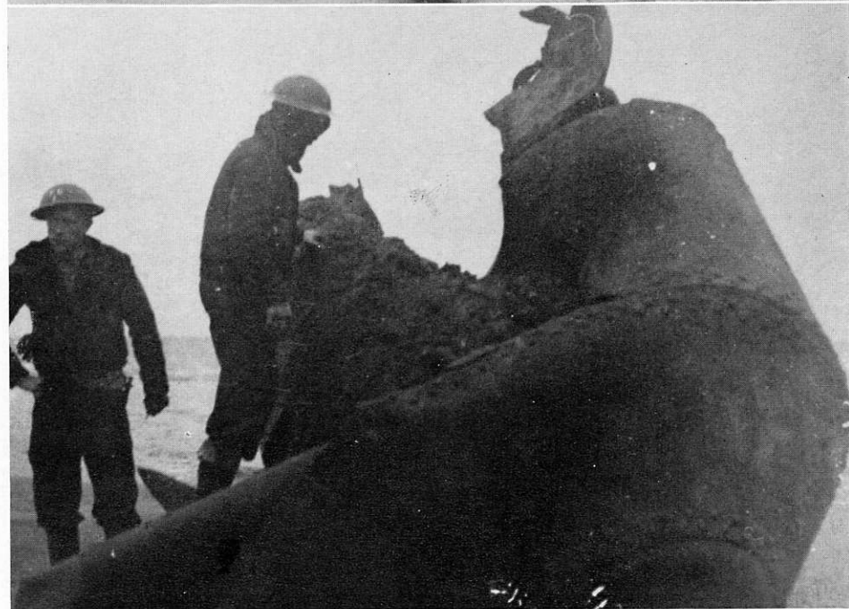
Before and After: In the upper photo the Crusader's demolitions party makes a start on getting rid of the buoy which drifted ashore on the Korean island and became half-buried in sand. To begin with they used plastic explosive and with it blew away the exposed part of the buoy. The lower shot shows a portion of the buoy after it had been blown clear of the sand by a 25-pound charge of amatol. The photos give some indication of the conditions under which the job was carried out. (CU-343 and 351).
