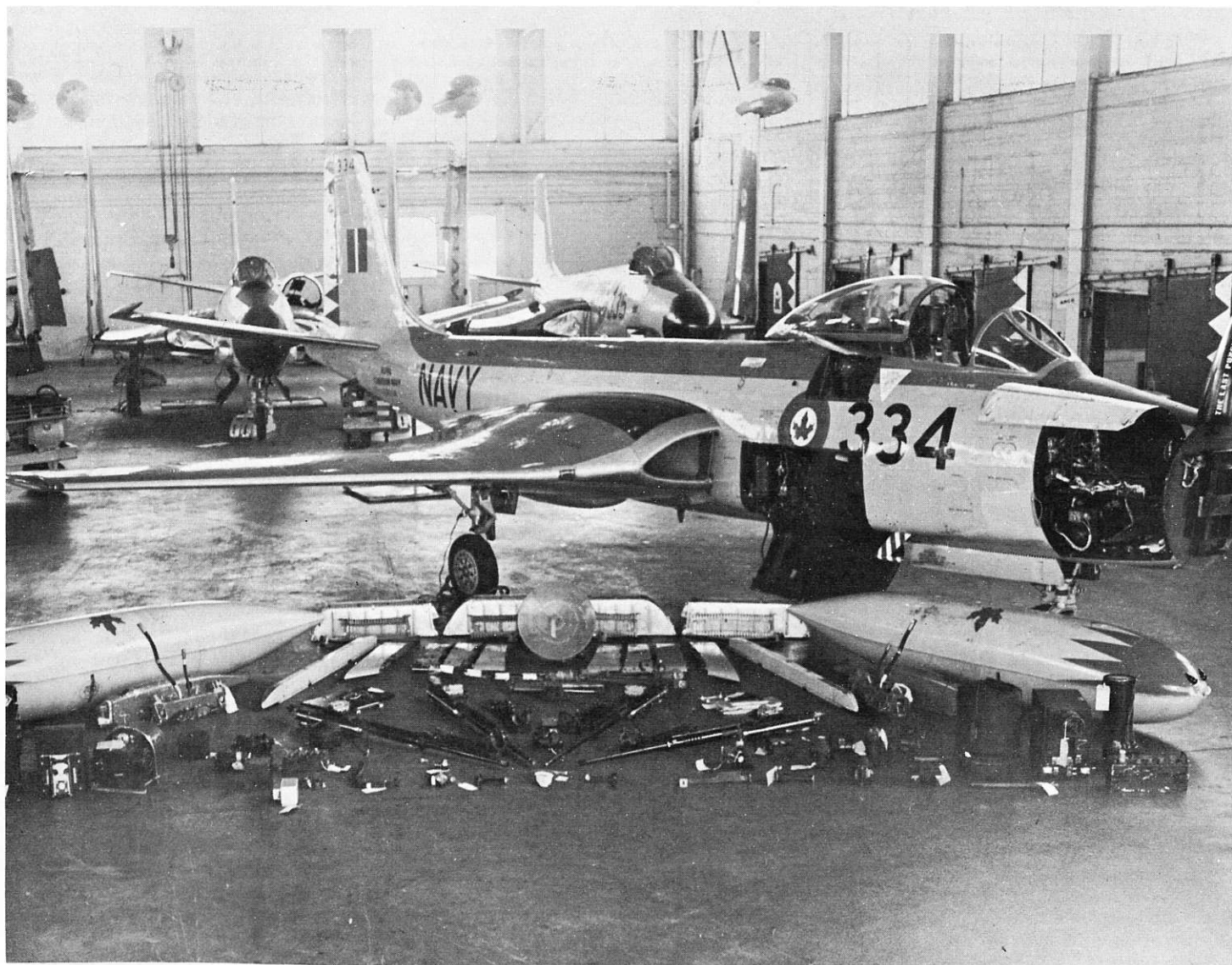
More than half a ton of fighting and other gear was removed from Banshee 334 to prepare it for its flight to the Southern Alberta Institute of Technology at Calgary. The picture shows the equipment removed and some of the ballast weights that were installed to assure normal flying. (DNS-29528)
