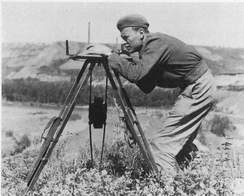
Corporal M. A. Brodsky of London, Ontario, and Ottawa, is pictured plane tabling during a survey on the Hudson Hope Road at the Peace River and Half Way River, 36 miles west of the Alaska Highway at Fort St. John. (Canadian Army Photo WC-634.)
