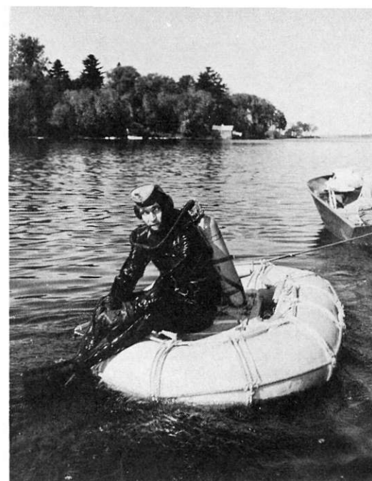
Ord. Lt.-Cdr. G. D. Cook tests the sea-worthiness of a new fiberglass Carley float built in HMC Dockyard, Esquimalt. The float is rot-proof and unsinkable. (O-6005)
